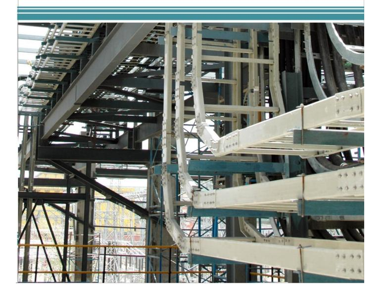
SATYAM Make FRP Ladder Type & Perforated Type cable tray gives the good support to Electrical Heavy Cables & Instrument Light Cables respectively mainly in chemical Industries or any corrosive Atmosphere. The Cable trays are manufactured from the polyester resin system with Fire Retardant & Ultra Violet resistant Properties.
